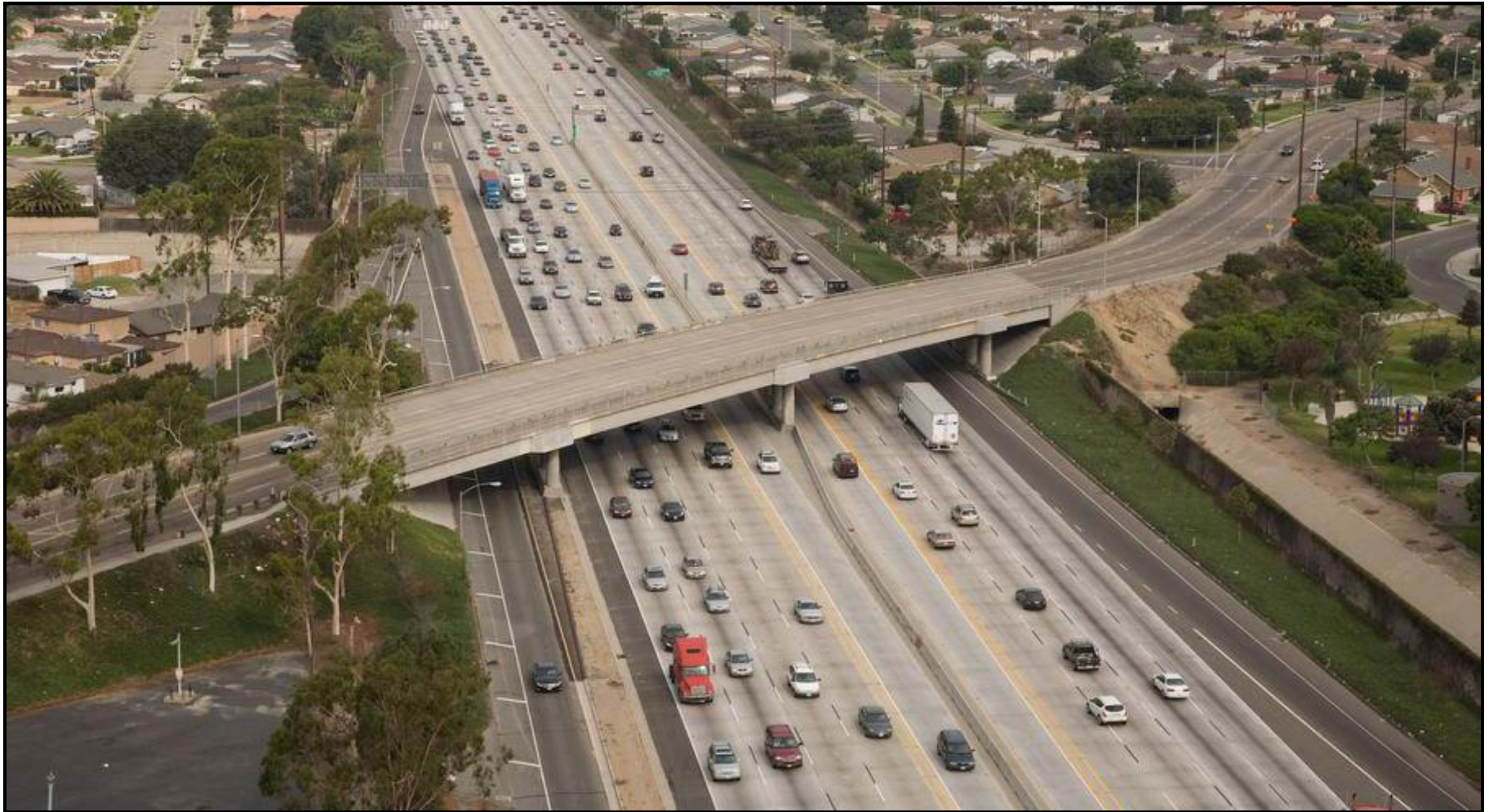
I-405 looking northwest at Springdale Street overcrossing
